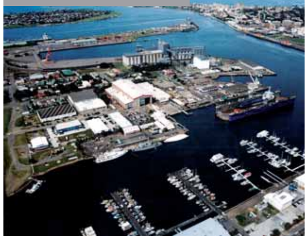
Refit work underway
